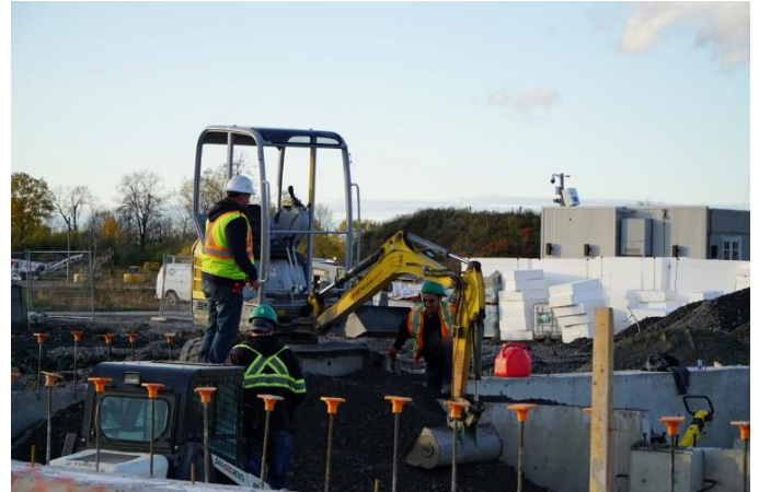
Work in progress at the building site
