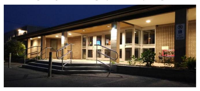
The steps, columns, front doors and vestibule and front canopy ceiling and lighting at the front entrance have all been replaced. The exit doors from the lounge were also replaced and an access ramp installed.
